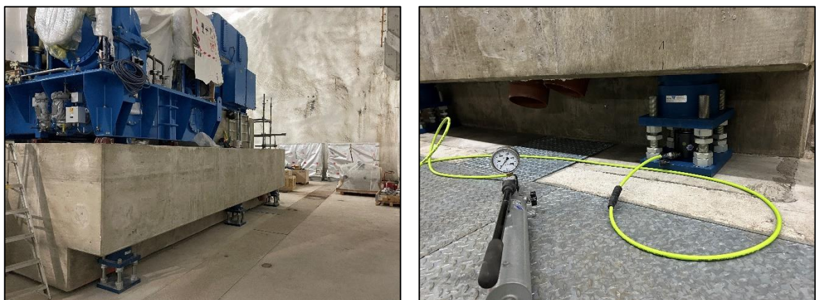
Figure 1.3: Installation of the Spring Elements / Lifting of the Foundation
